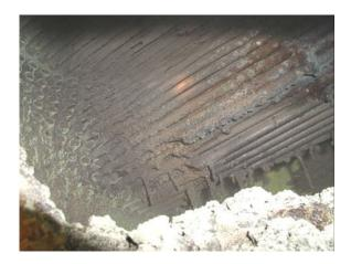
Figure 12. Damaged reheater tubes
