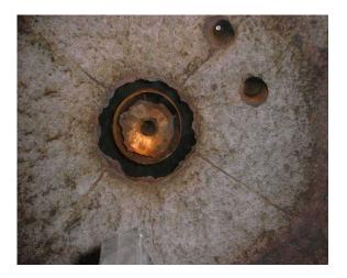
Figure 1. Burner throat showing backfiring
