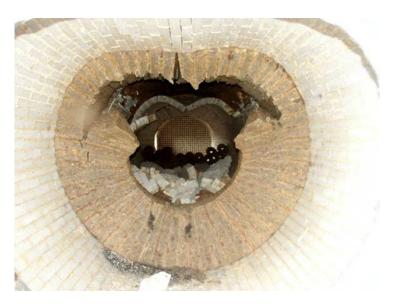
Figure 3. Caved in refractory
